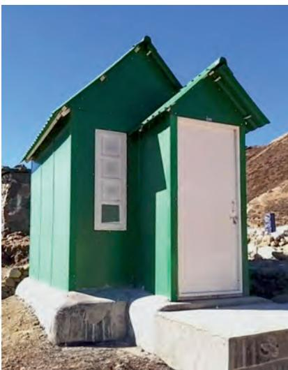
**We also conducted field trials with the Indian Army's Eastern Command at Bumla Pass to evaluate the thermal insulation properties of composite-based porta cabins at altitudes over 15,000 feet.**
